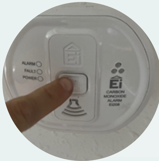
Testing a CO alarm
