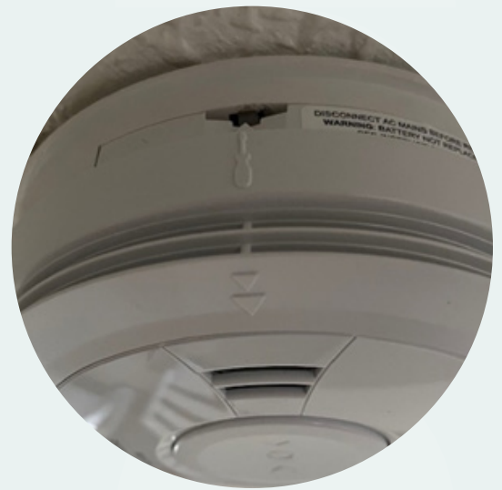
Removal slot indicated by the screwdriver icon
