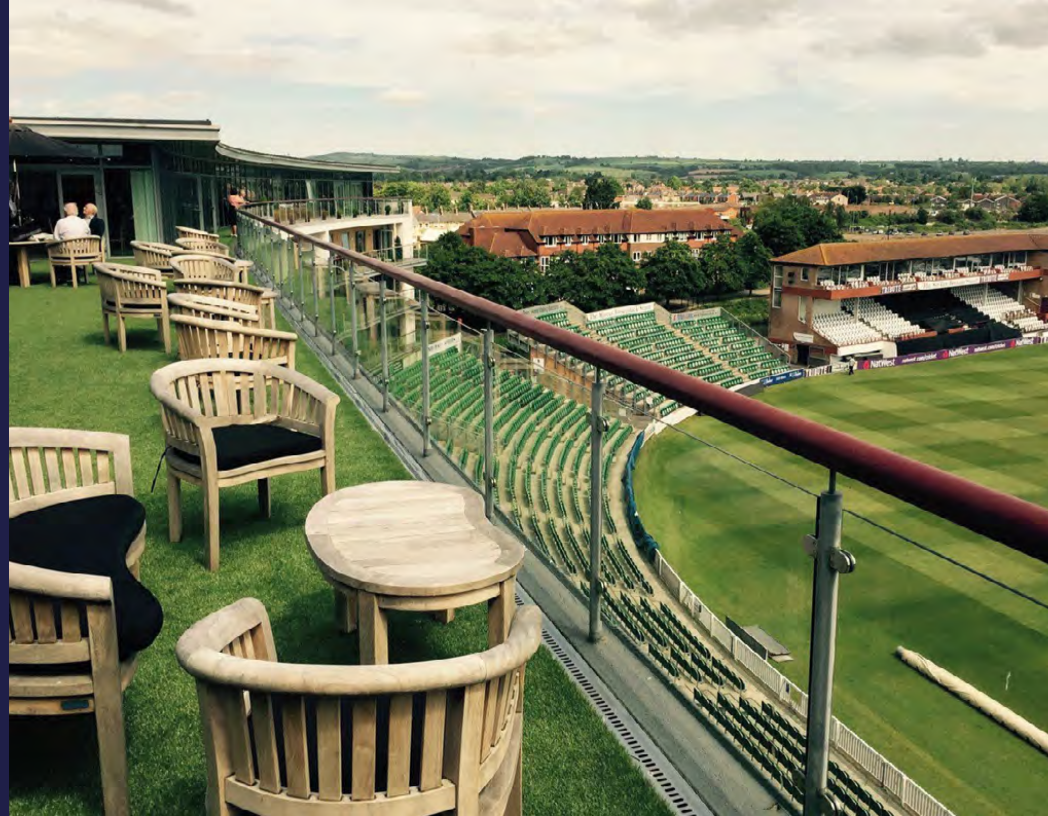
Senior housing development built as enabling project for new stand at Somerset County Cricket Club in Taunton.
