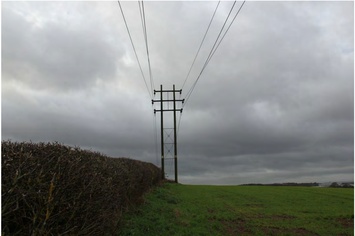
Photo 9 Temporal parcel looking west.
