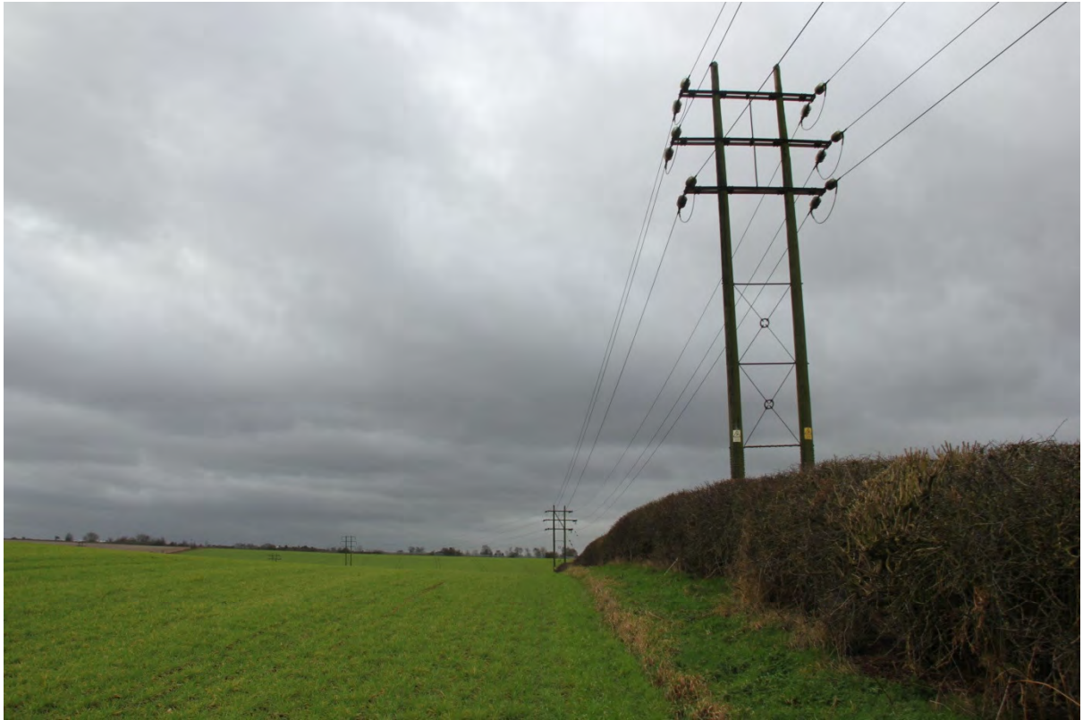
Photo 11 Temporal Parcel looking west.
