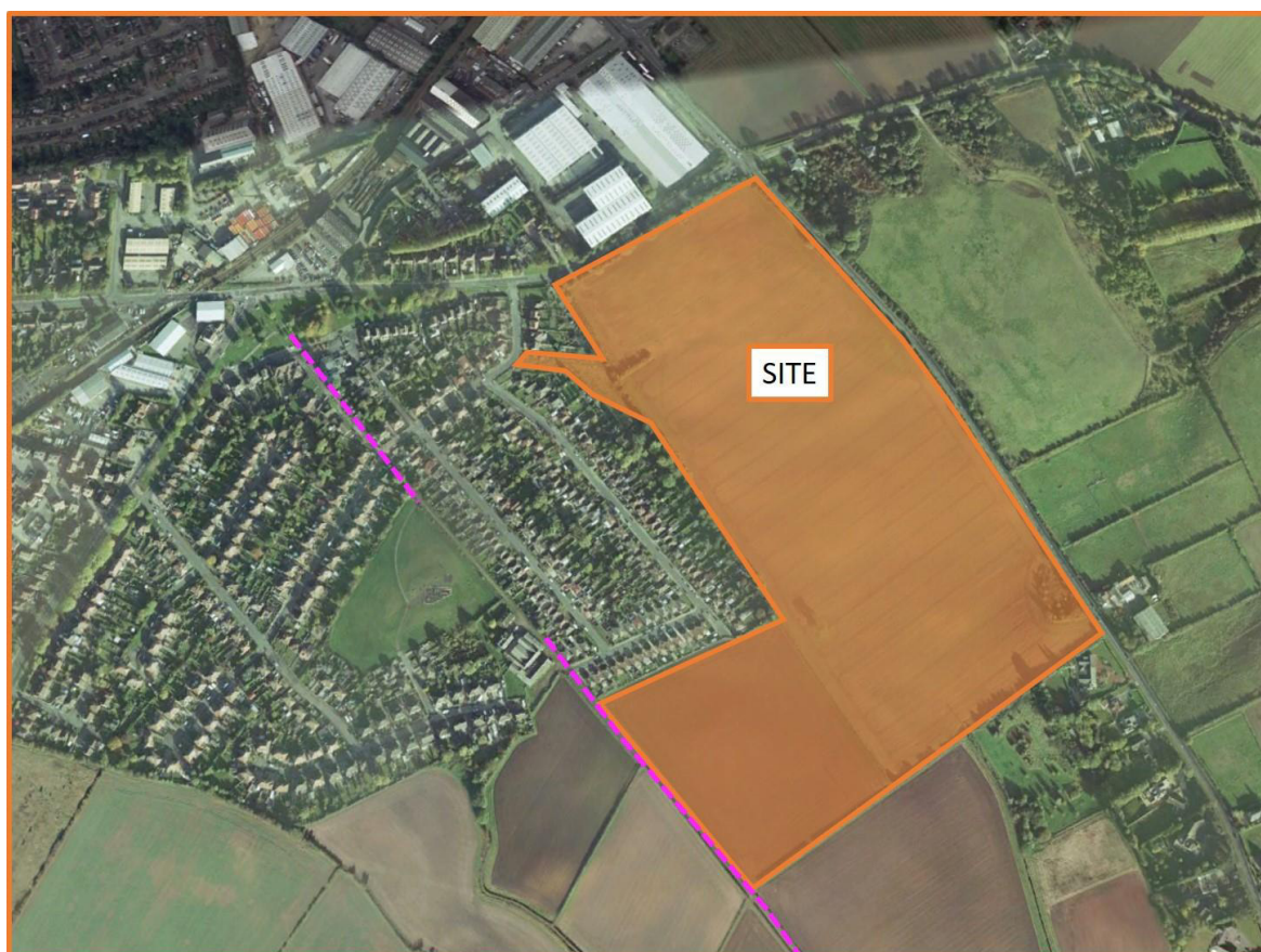
Figure 3: aerial photograph (indicative site boundary)
