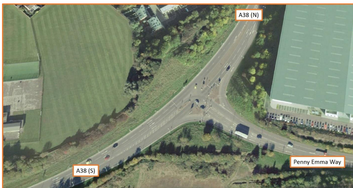
Figure 9: existing A38/Penny Emma Way junction
