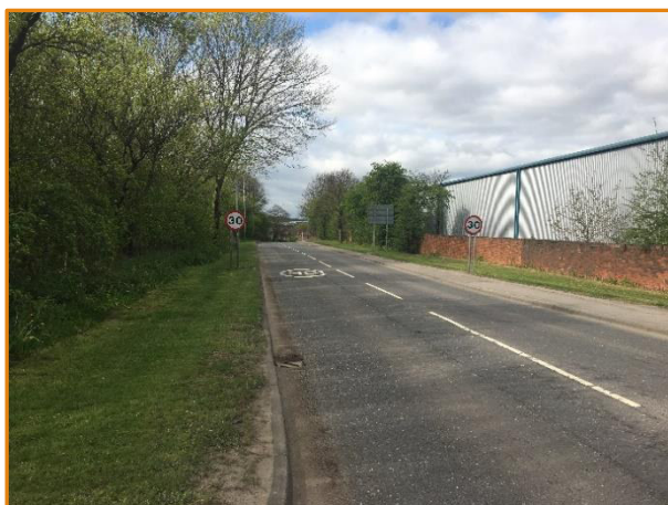
Photograph 1: footway on Newark Road (looking west) along site frontage
