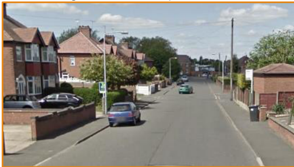
Photograph 5: footways on Farndon Road
