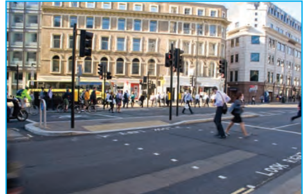
Staggered signalised crossing without guardrail
