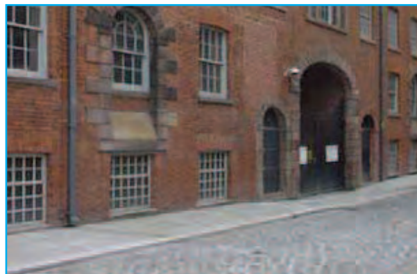
Access to commercial property with limited visibility.
