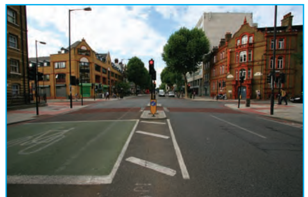
Traffic signal junction with clear and simple pedestrian crossings and advance cycle stop lines. Note lack of guardrailing and buildings close to junction corner, and tight corner radii.
