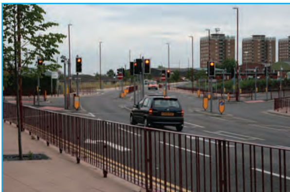
Newly-implemented highway scheme with extensive guardrailing
