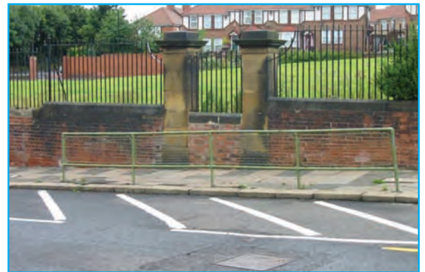
This guardrail has no function - the pedestrian route it was protecting has been closed - and can therefore be removed.
