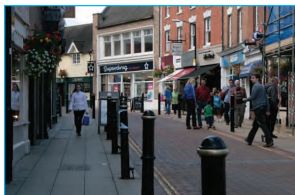
Bollards can add considerably to street clutter.
