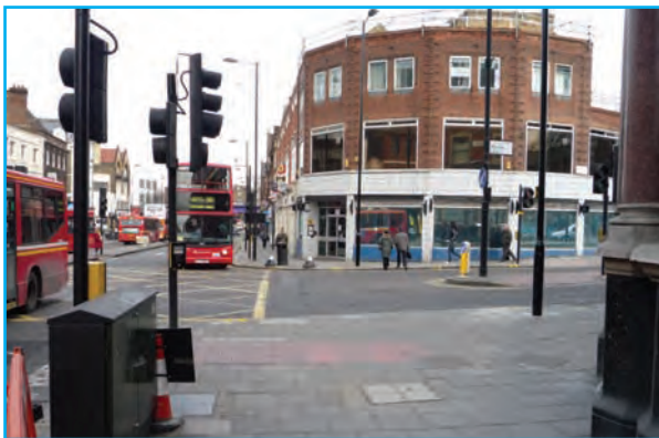
Mare Street Hackney - Before and after a decluttering scheme in August 2007. Casualty records have revealed a safety neutral outcome.
