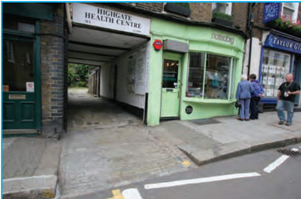
Footway crossover access to commercial premises
