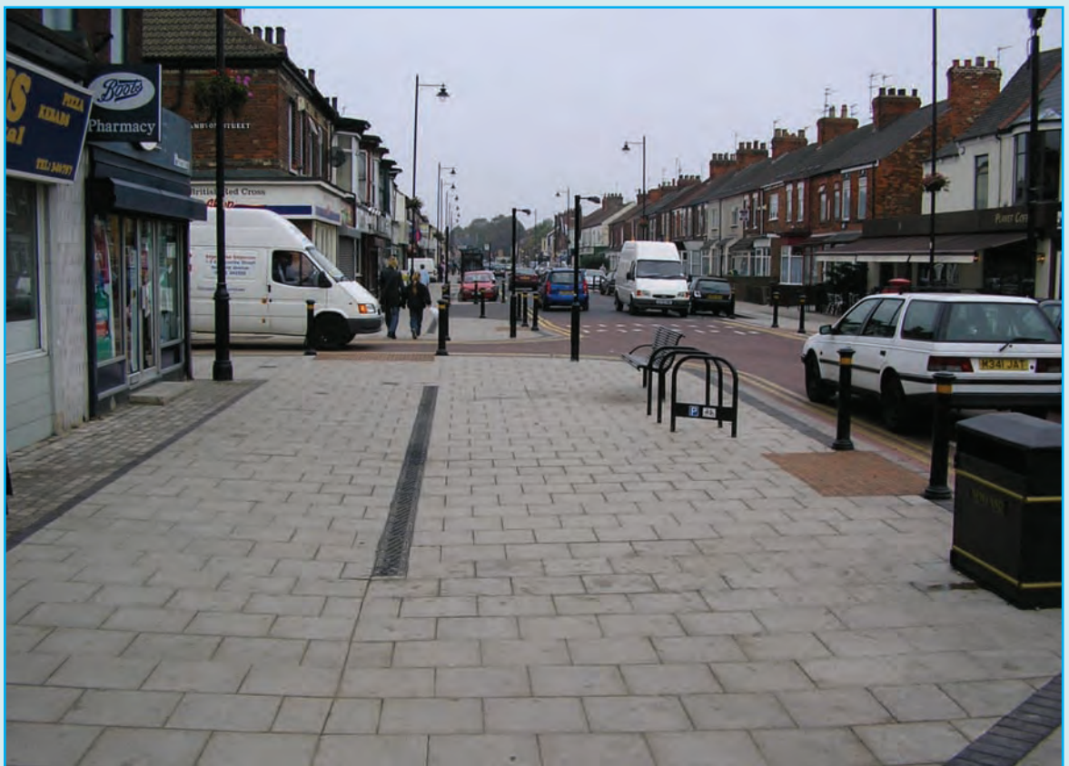
Footways widened significantly by narrowing carriageway
