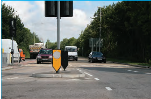
Keep left bollard, with rear face uncoloured
