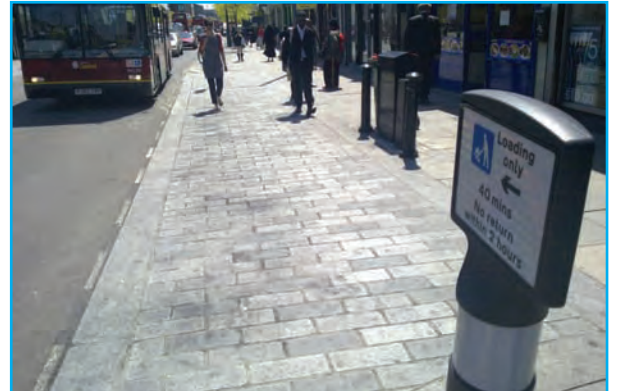
On-footway servicing bay - Walworth Road MPR Scheme, London
