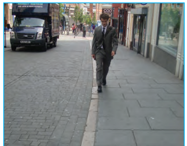
Kerb heights of between 75mm and zero (at informal crossings) were used with streetscape improvements in the centre of Nottingham.
