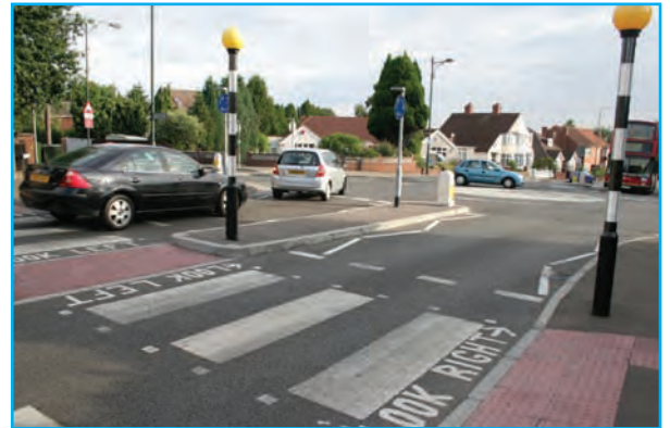
Zebra crossing located close to road junction.
